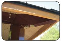
**Options Shown:** 2x6 Tongue & Groove Roof Decking, Steel Post & Beam, Roof Decking modified for Skylights\*\*
