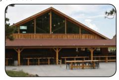
**Options Shown:** 12x12 x ¼" Steel tube posts, 12x12 x ¼" Steel tube header beams, Glu-Lam beams & traces, 2x6 T&G roof
